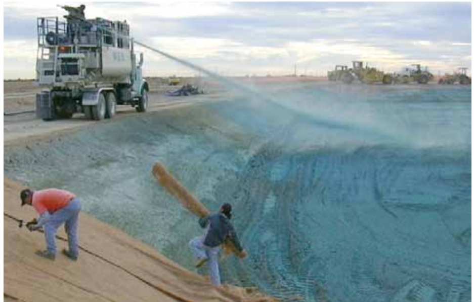
This truck is spraying EZ Bond Maximum Fiber Matrix to temporarily stabilize dirt piles on construction sites. Phoenix Paper Products, the manufacturer of this paper and corn fiber product, received a loan from Upper Illinois River Valley CDC, a multibank CDC in north central Illinois.
